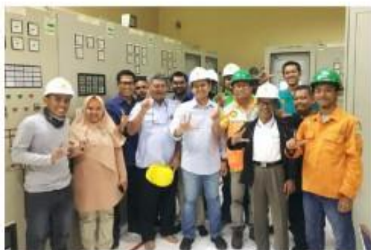
Successfully charging completed in 150KV Substation in Sulawesi at Indonesia
