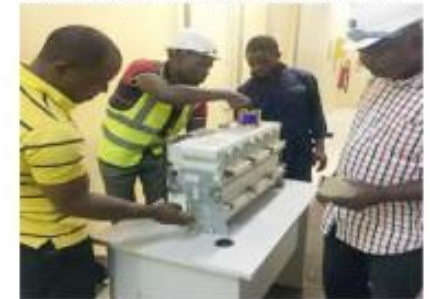
Shutdown Maintenance of LT Breakers for M/s. PZ Wilmar
