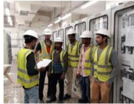
132/11kV Bu Gam Substation
