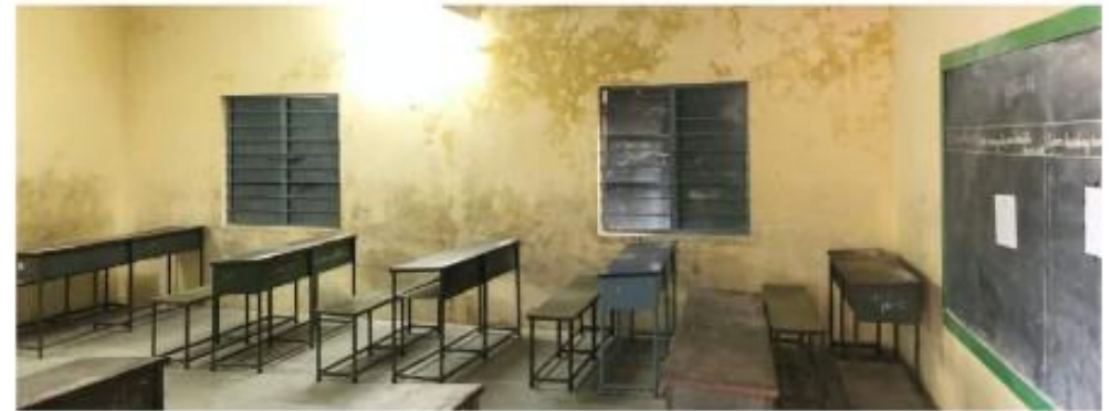
Classrooms with lights & fans provided by Voltech
