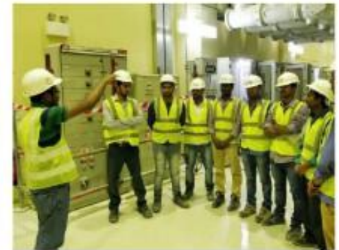
400/220/132/11kV Doha south super Substation
